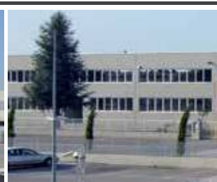
REMER ENGINEERING 2 high-tech production.
